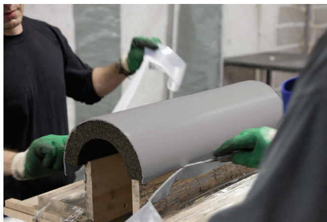
Terostat PC® FRI pipe shell application
